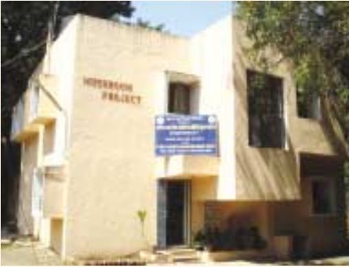
Fig. 1. AICRPM Centre, Pune
